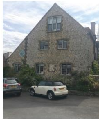
Tythe Barn, 18th century, listed building
