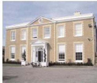
Ovingdean Hall, Listed building
