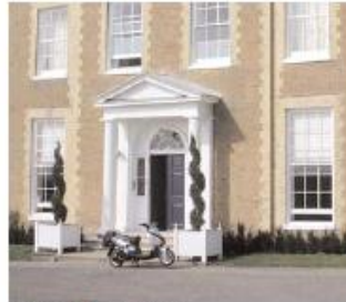
Ovingdean Hall, Listed building
